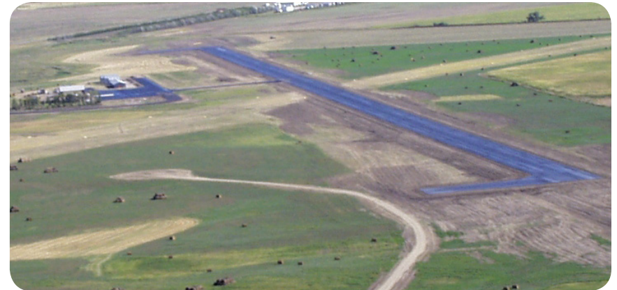
New Runway 12/30 at the Chamberlain airport
