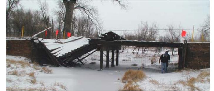
An example from Tripp County is pictured, but it is not the only case. In the past two years alone, six county bridges had to be completely replaced because of damage from illegally overweight trucks:
