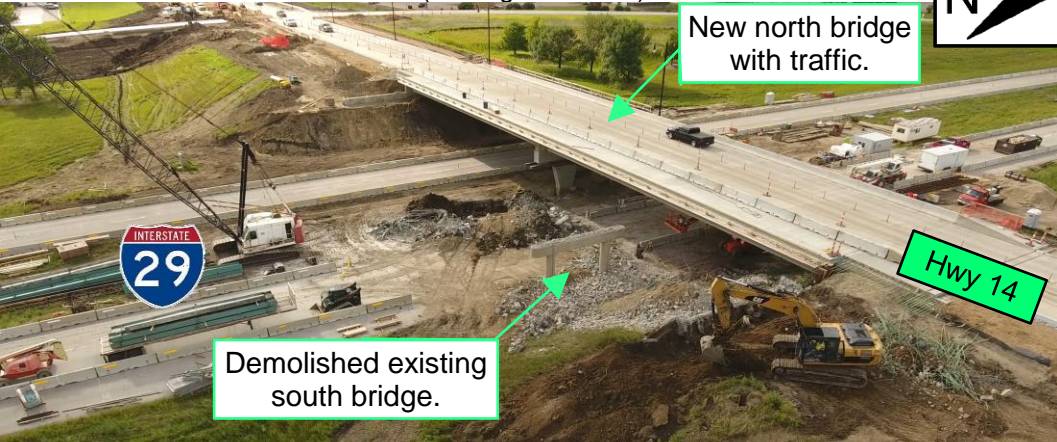
Project Photo: The demolished south bridge @ I-29. (looking northwest)
