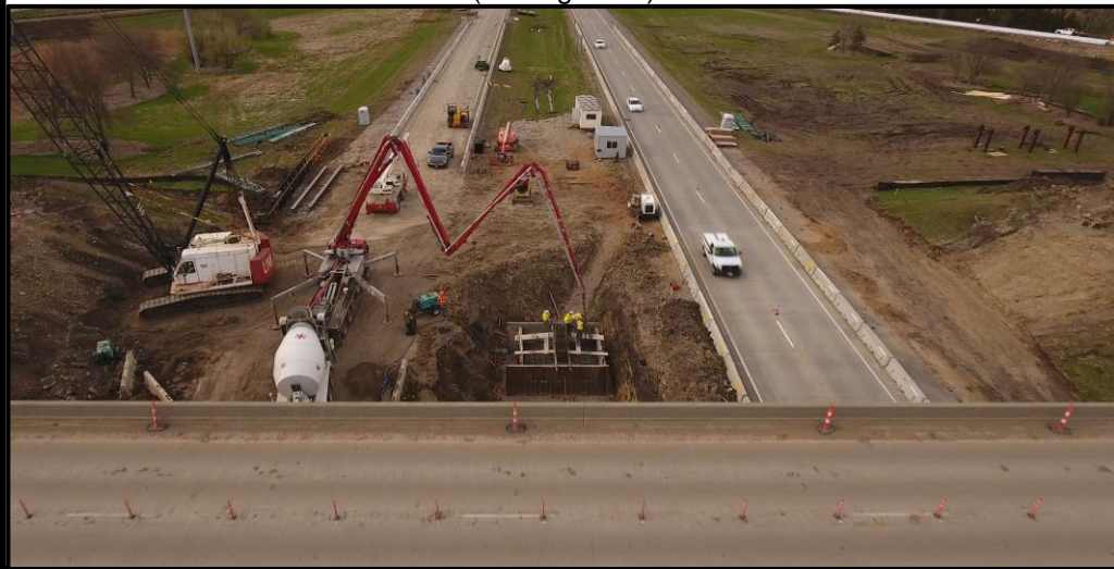
Project Photo: Installation of the foundation for the I-29 median bridge bent (looking north)
