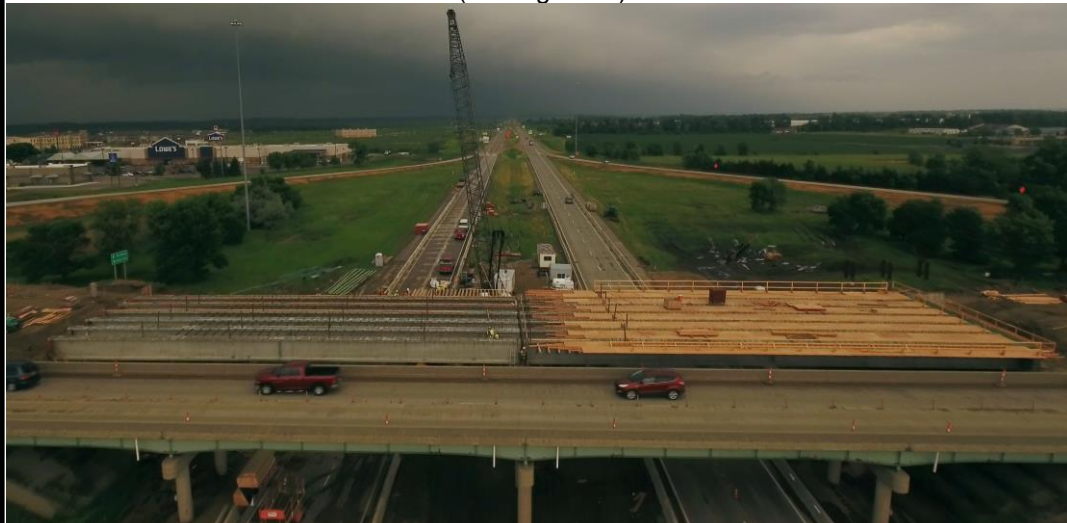
Project Photo: Bridge decking work @ the new I-29 bridge (looking north)
