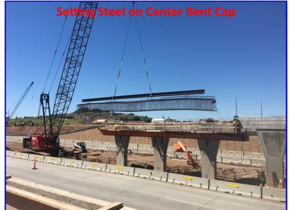
Setting Steel on Center Bent Cap
