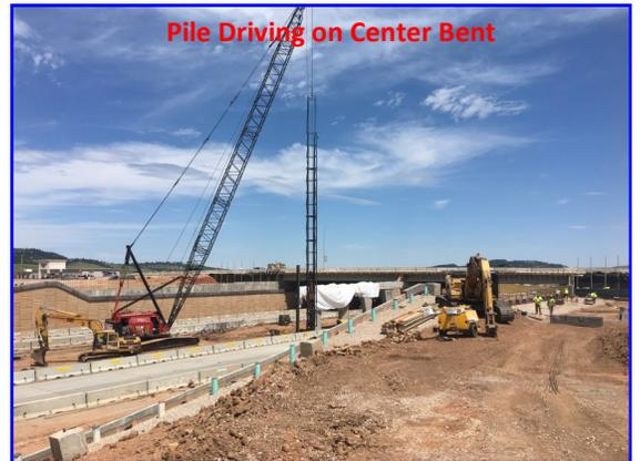
Pile Driving on Center Bent
