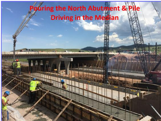
Pouring the North Abutment & Pile Driving in the Median
